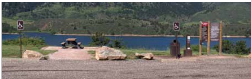
ADA upgrades on the east side of Horsetooth Reservoir Photo: Steve McCorkel
