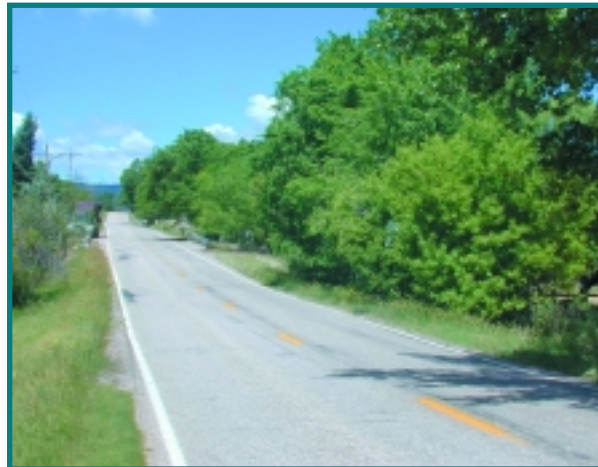
Vegetation overgrowth can cause hazardous traffic conditions. Can you find the speed limit sign in this picture?
